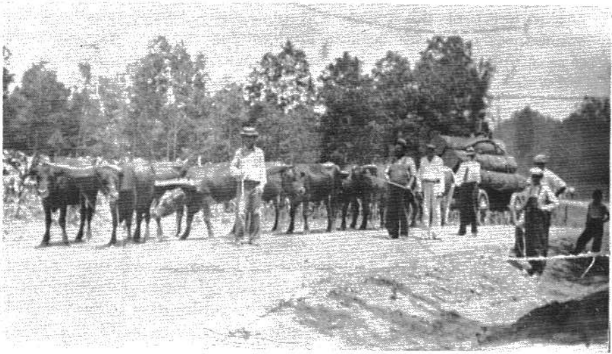
Work crew uses oxen to clear land at the Skyline Farms project. Photograph provided by Mrs. Ruth Harrington.
